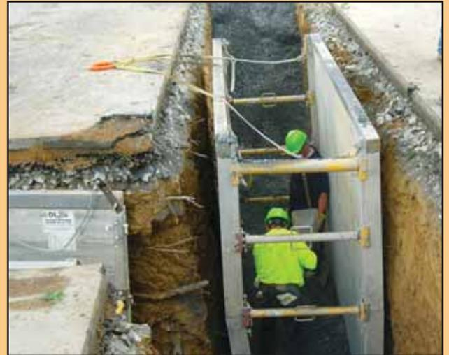
**UPGRADING INFRASTRUCTURE** — Township crew works on replacing 300 feet of sewer line on Gale Road. The project, which also included installation of six lateral lines, was done at approximately half the cost because of the use of the Township Public Works Department work force.
